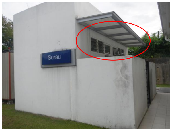
Figure 4. Surau 11 with high vents and ablution space provided in walled area outside prayer space.
